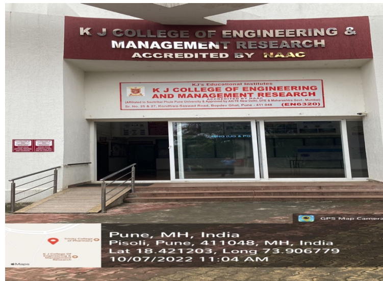
Ramp with metal railing at the entrance
