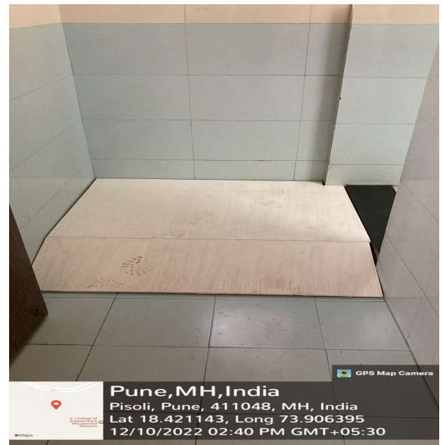
Ramp at toilet block entrance
